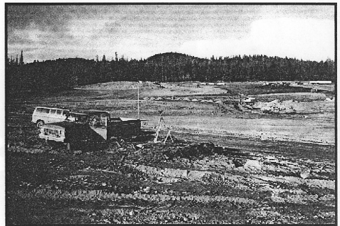
Mount Polley plant site preparation - September 1995.
