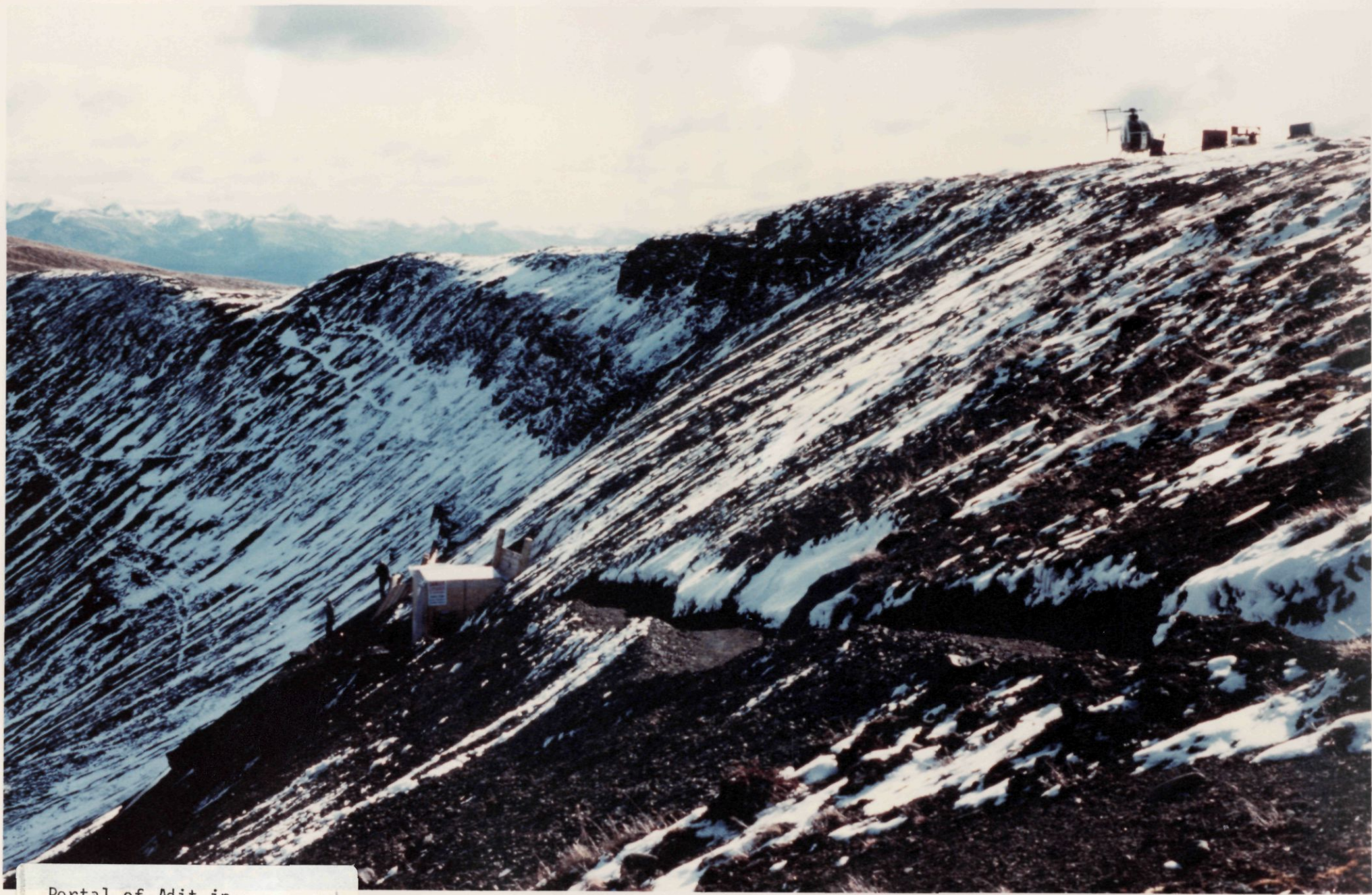
Portal of Adit in Lost-Fox Pit
