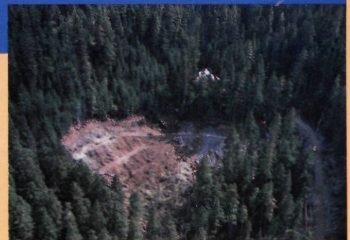
TUNNEL PORTAL SITE PREPARATION.
