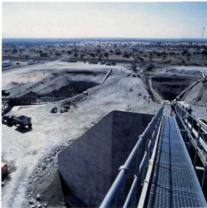
Construction at the US$200 million Bafokeng Rasimone project, South Africa
