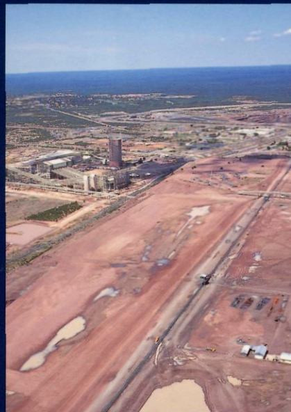
A recently completed expansion programme has doubled capacity at Orapa Mine in Botswana
