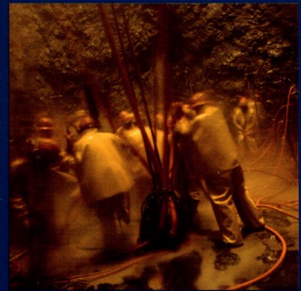
Shaft sinking operations at Vaal River Operations, South Africa
