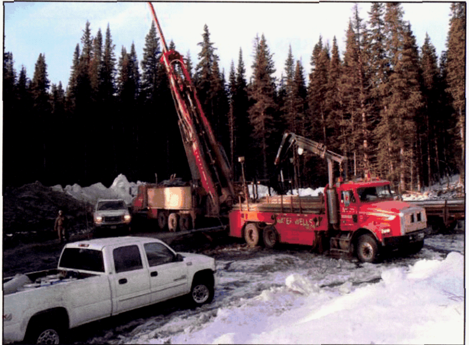
ANGLE DRILL HOLE AT LOSSAN PROJECT FEBRUARY 2005
