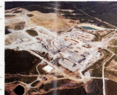
Gibraltar Mine. Taseko plans to reopen Gibraltar, mining 35,000 tonnes/day with an innovative, high efficiency copper refinery on site.
