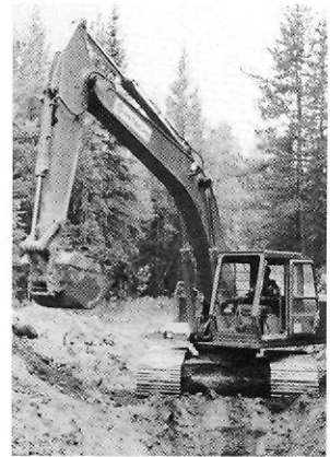
Excavator trenching on Nation River's property near Fort St. James, August 1987.
