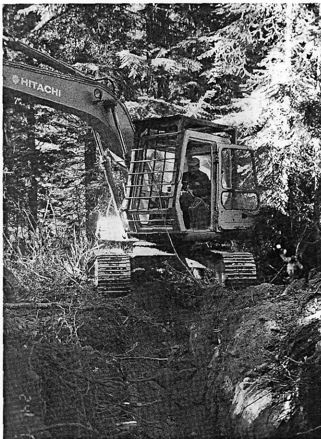
Excavating the discovery trenches on the Gold Mountain zone.
