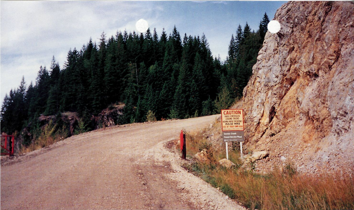
MAIN ACCESS ROAD FROM HIGHWAY 23 LEADING TO THE J & L SITE.
