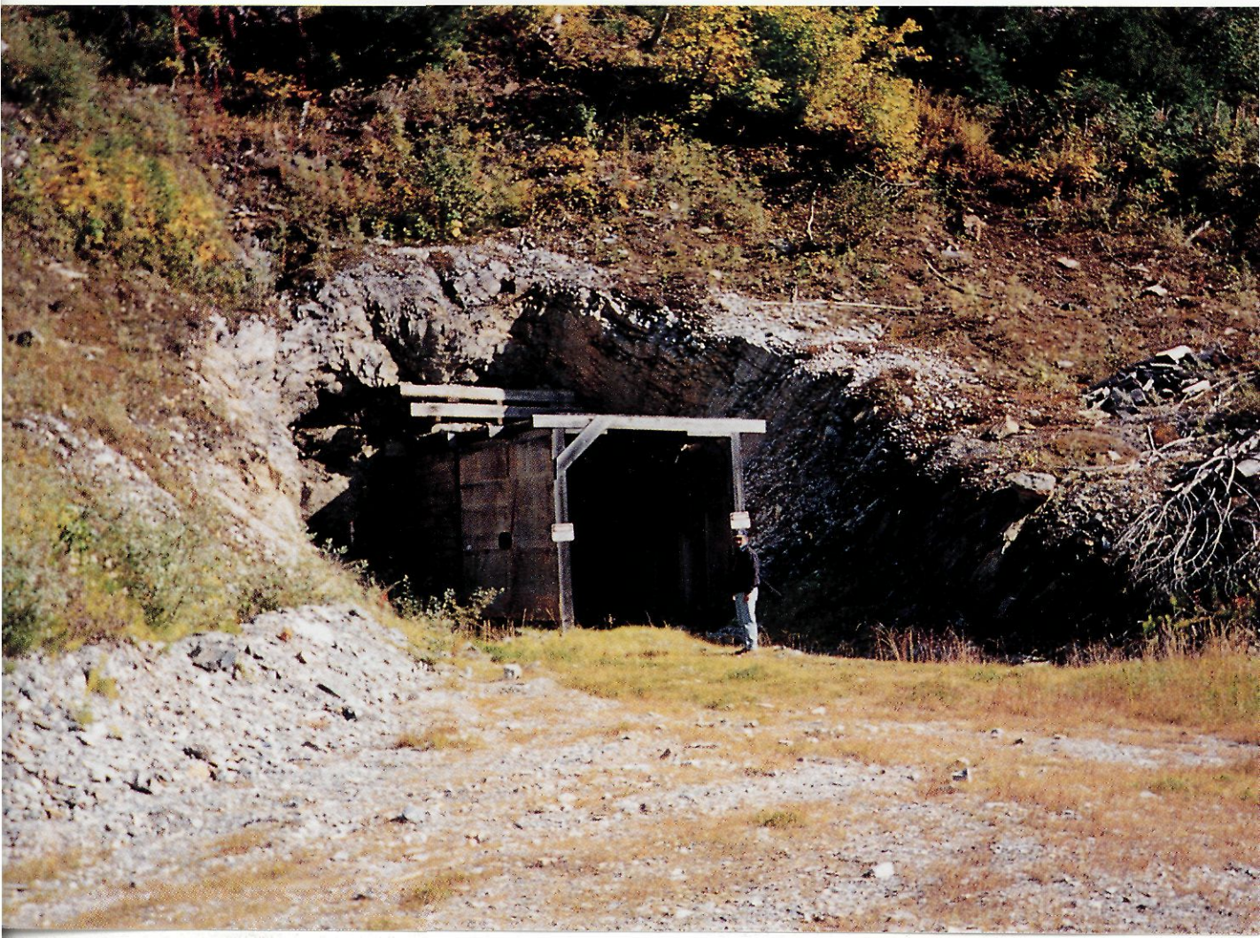
830 METRE LEVEL TRACKLESS PORTAL, ONE OF THE OPENINGS TO THE UNDERGROUND WORKINGS.
