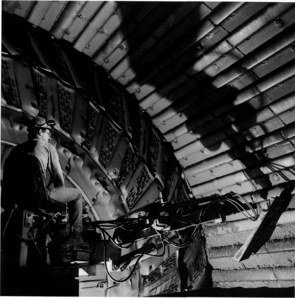
John Seymour, lining machine operator, relines the inside of one of the large semi-autogenous grinding mills.
