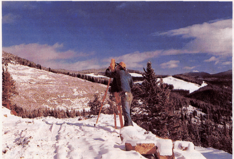
Surveying the central pit area with electronic distance measuring equipment.
