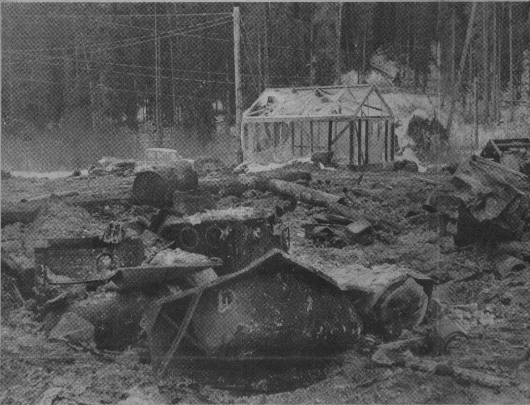
BLACKENED REMAINS show the savage destruction which can result from a house fire. This used to be the Topley
