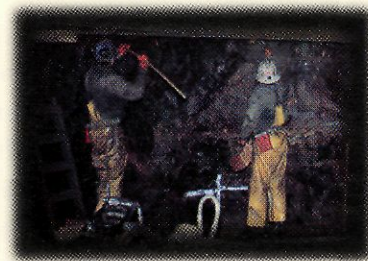
Wheaton River re-opened the underground operations during the summer of 1993.
