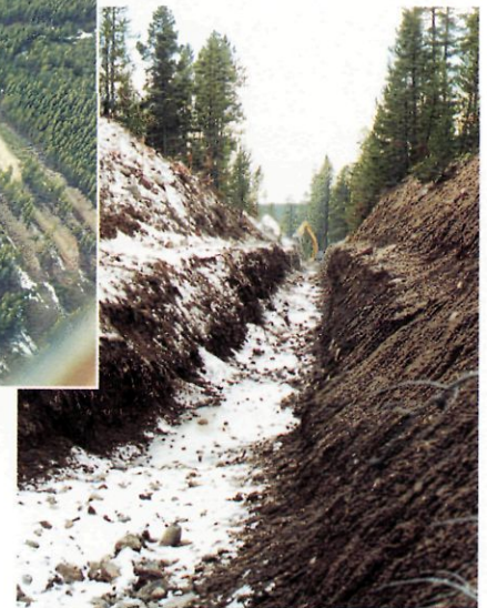
Getty South Trench
