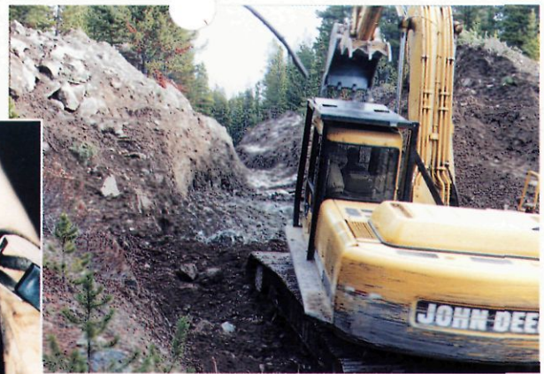
Getty South Trench
