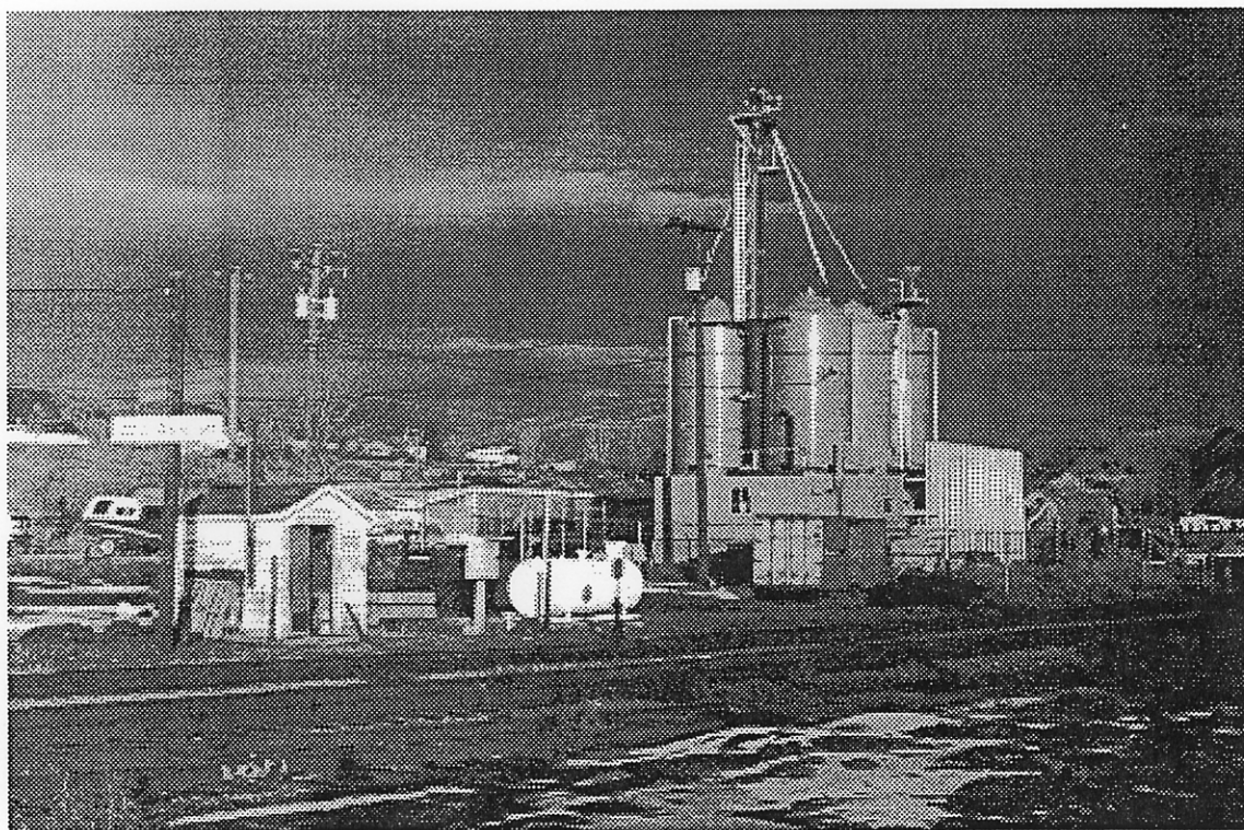
Figure 8. New zeolite processing plant and storage silos of C2C Mining Corp. at Ashcroft.
