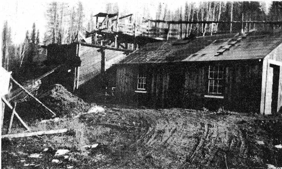
Ore chute and Blacksmith Shop, where Tom Haig and Ridsdale sharpened the drill steel. Photo courtesy John Bovill
