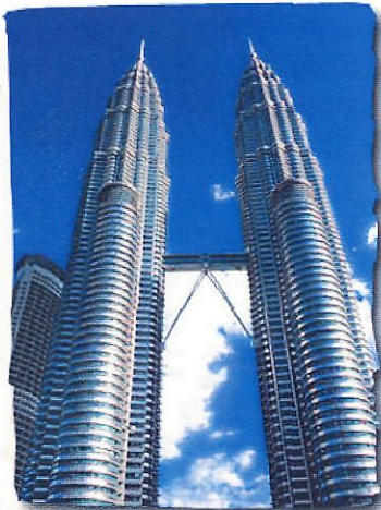
Molybdenum alloys clad the Petronas Twin Towers in Kuala Lumpur, Malaysia, among the world's tallest buildings.
