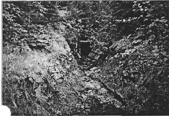
Windpass portal and drainage
