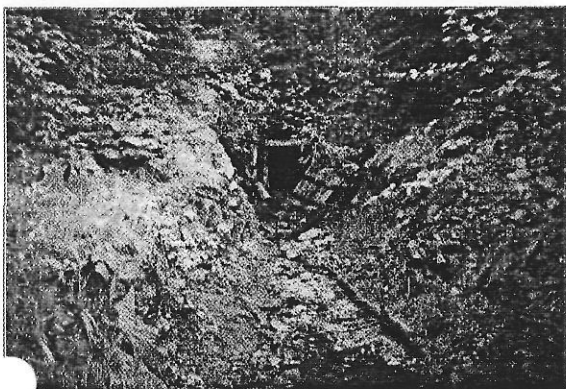
Windpass portal and drainage
