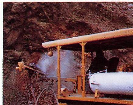
A drill rig prepares the face of the upper Howard drift for blasting.
