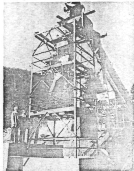
Bulk sampling plant designed to process 25 tons of gold ore per hour for feasibility studies at the B.C. property of Carolyn Mines Ltd.
