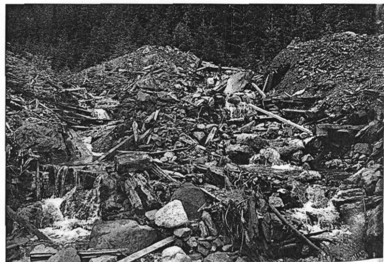
Elevated iron 2200 level drainage mixes with cleaner waters of Jane Creek and causes the precipitation of iron oxides both here and in Britannia Creek immediately below.
