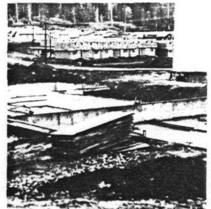
Re-activating Phoenix in 1956. Repairing workers' houses.
