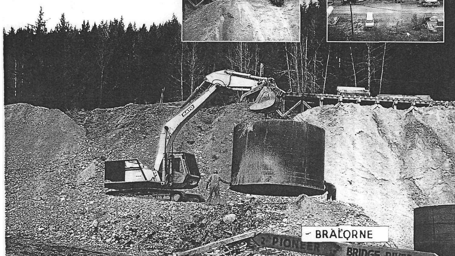
Construction of new mill facility is proceeding on schedule
