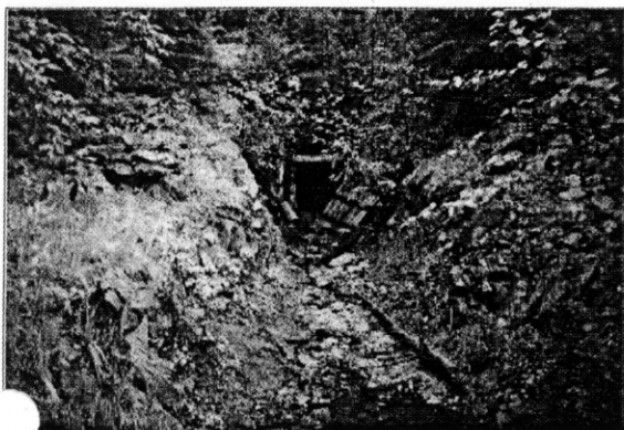
Windpass portal and drainage
