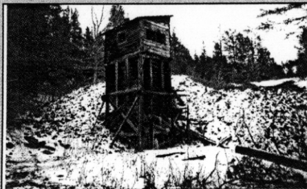
Windpass Ore sorting transfer
