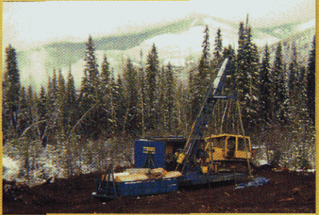
Initial drilling completed Nov. 1998
