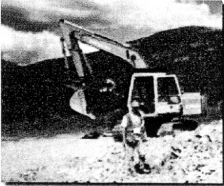
Trenching at McPhee
