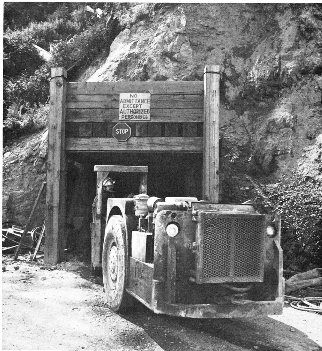
Scoop tram removing ore from main adit.
