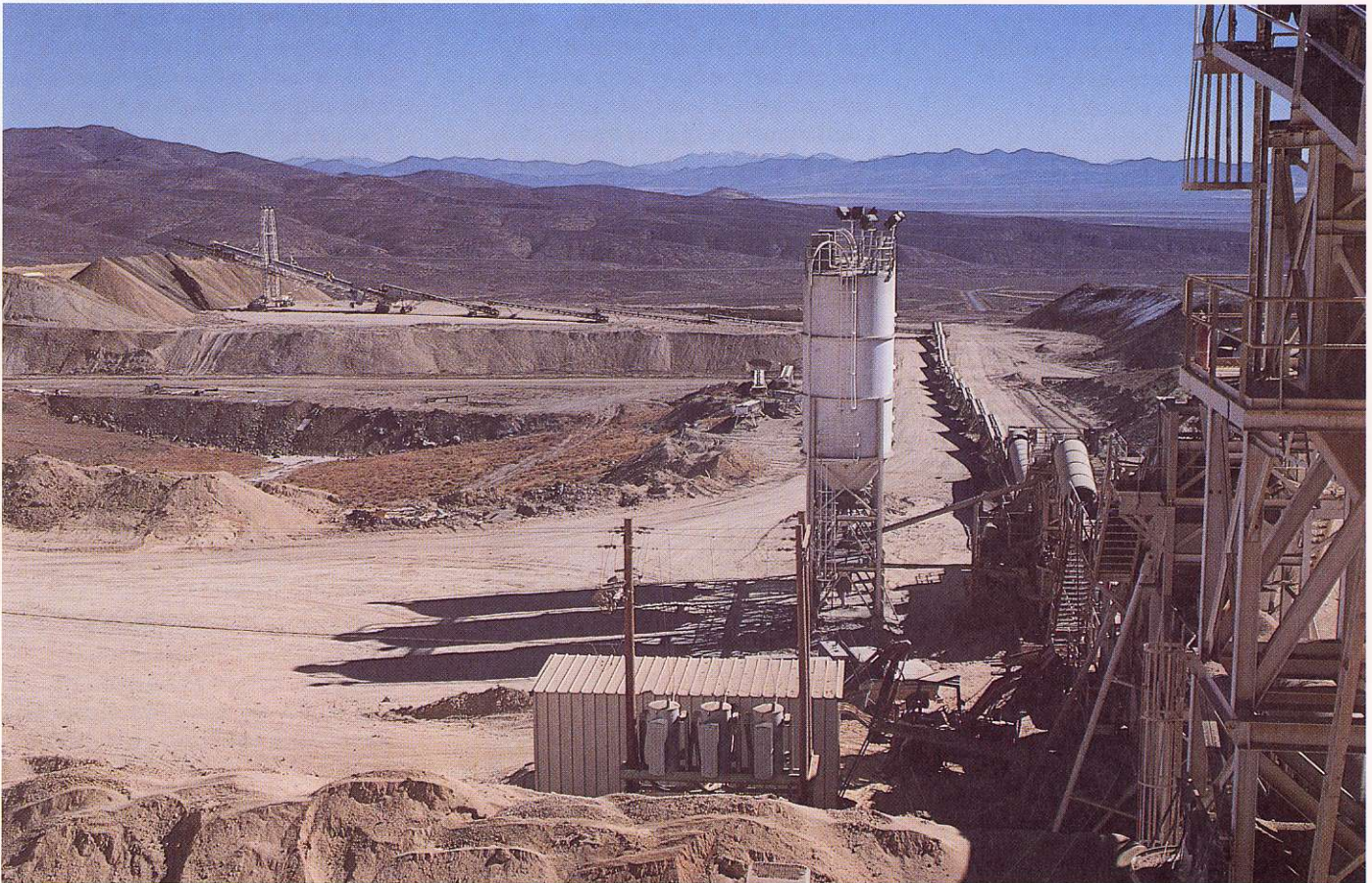
Stacking conveyors and leach pads at Buckhorn Mine.
