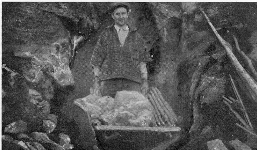
PORTAL OF MATILDA CLAIM TUNNEL, 1919
