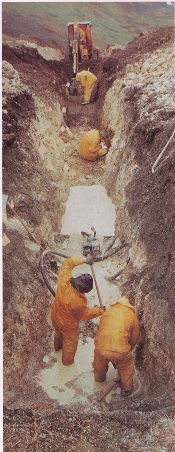
Typical Backhoe Trenching and Surface Sampling
