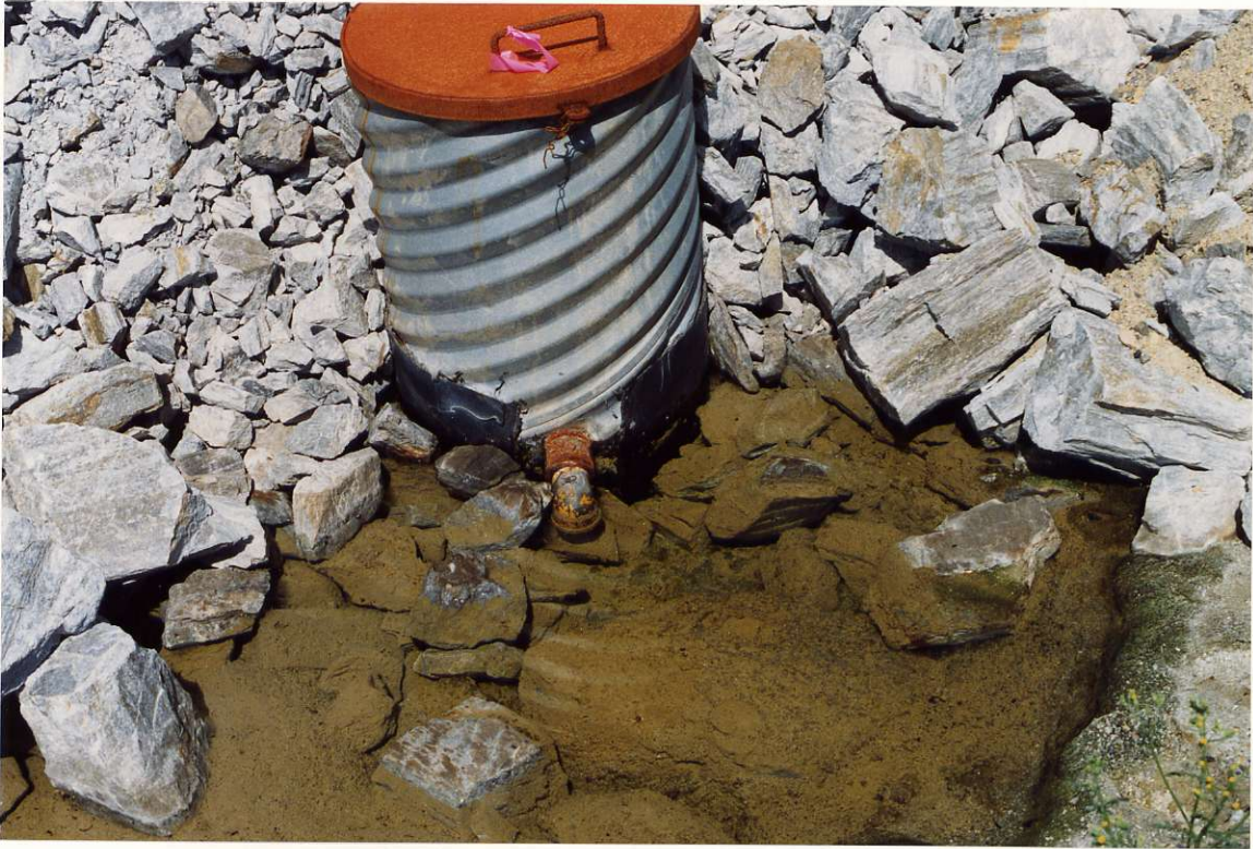
FIGURE 8: DRAINAGE CULVERT AT LOW CORNER OF WASTE/ORE PAD (JULY 27. 1989)
