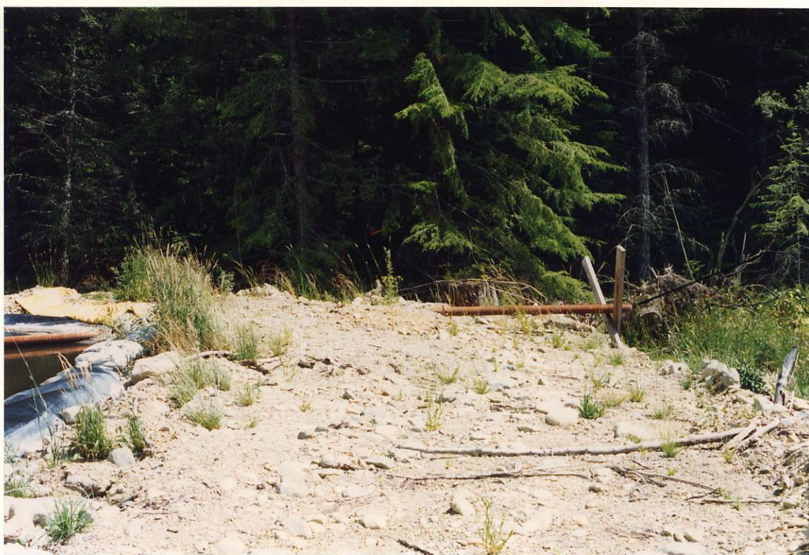
FIGURE 10: OVERFLOW DRAIN FROM MONITORING POND
