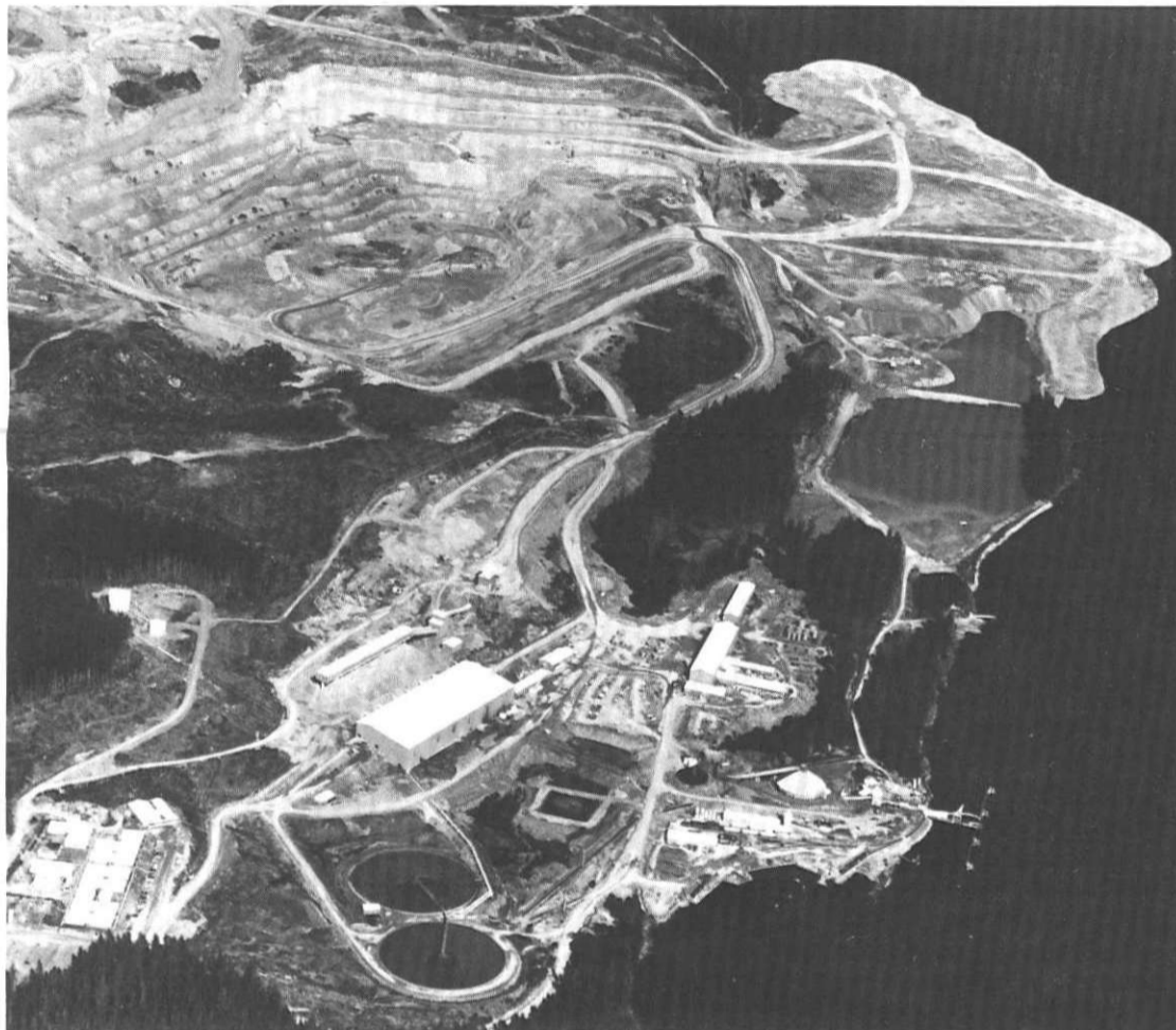
Aerial view of Island Copper's open pit mine near Port Hardy as it looks today. The pit eventually will occupy an area of about 490 acres.
