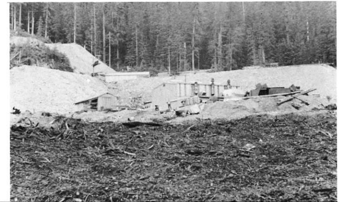
Looking north-east towards the diesel power house with the 1200 ft. level ore and waste dumps in the background.
