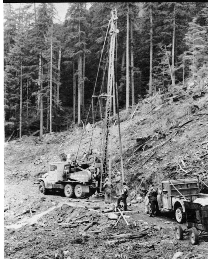
Drilling for foundation data at location of mill bins.
