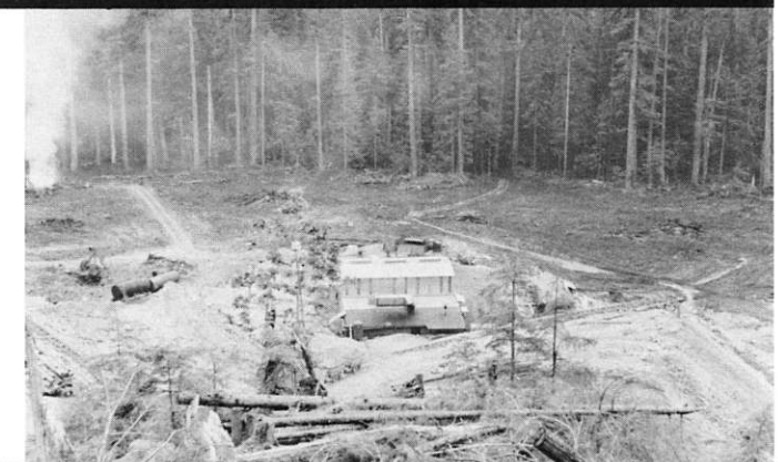
View of Power House and Lynx Site.
