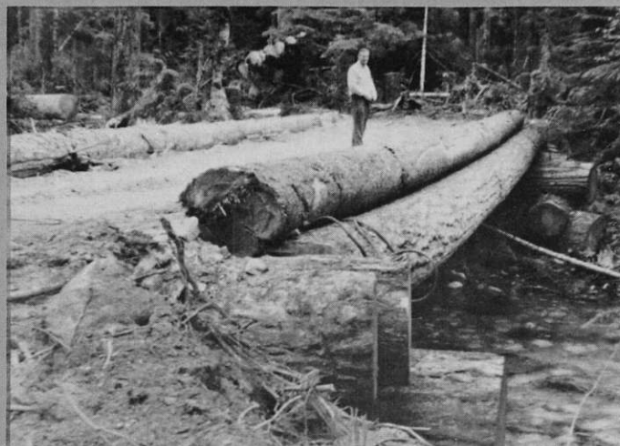
Bridge over Myra Creek
