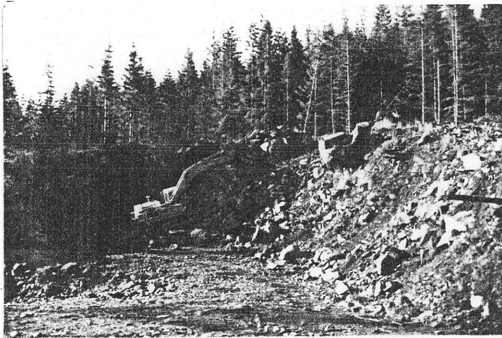
Figure 6. Trenching, Lake Showing.
