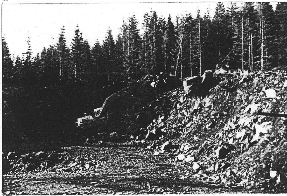
Figure 6. Trenching, Lake Showing.
