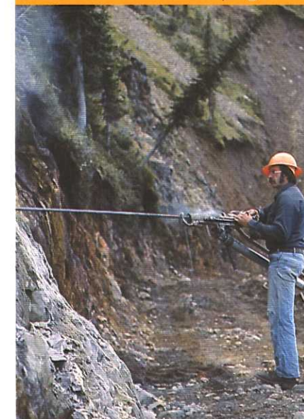
Surface Blasthole Drilling
