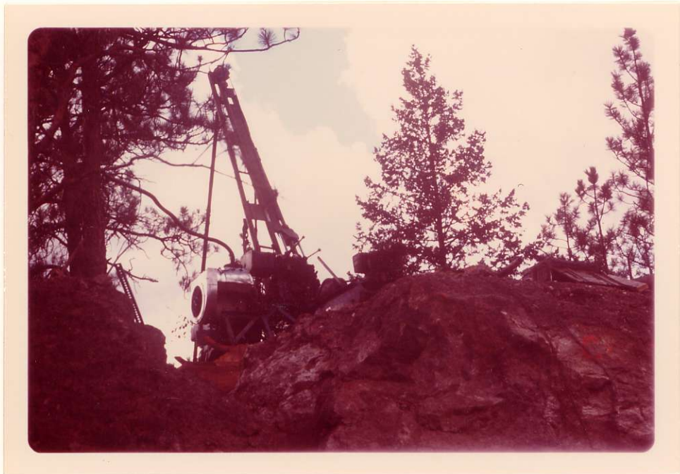
D. DRILL SET UP ON NO.1 HOLE
