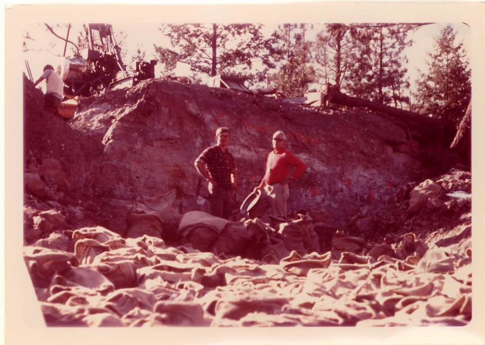
SACKED ORE SLASHED OFF FACE IN BACKGROUND D.DRILL SET UP ON #1 HOLE.
