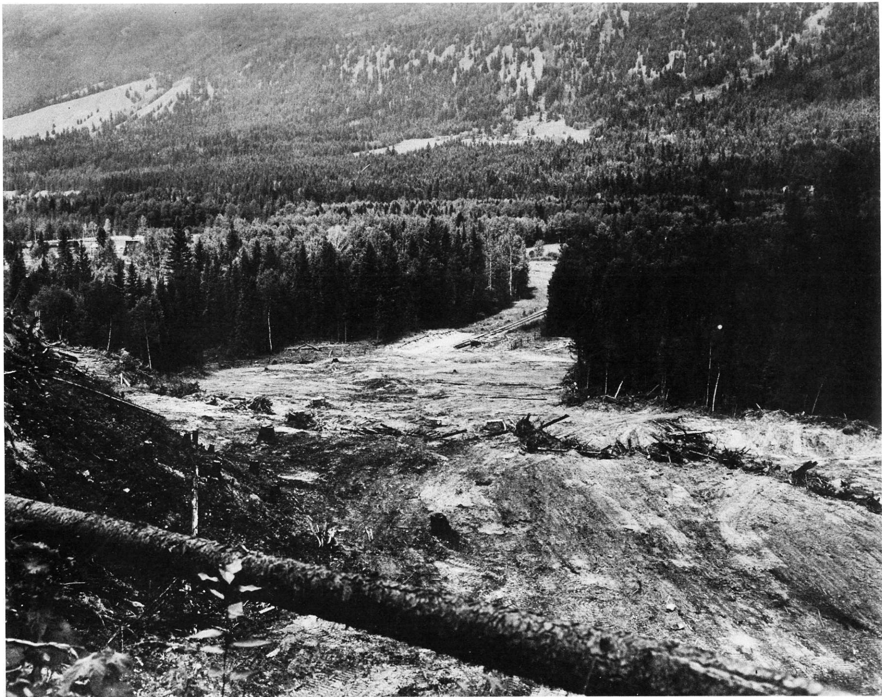
Rexspar plant and Mill Site cleared.
