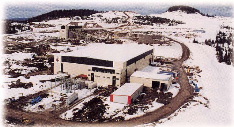
View of mill and concentrator buildings
