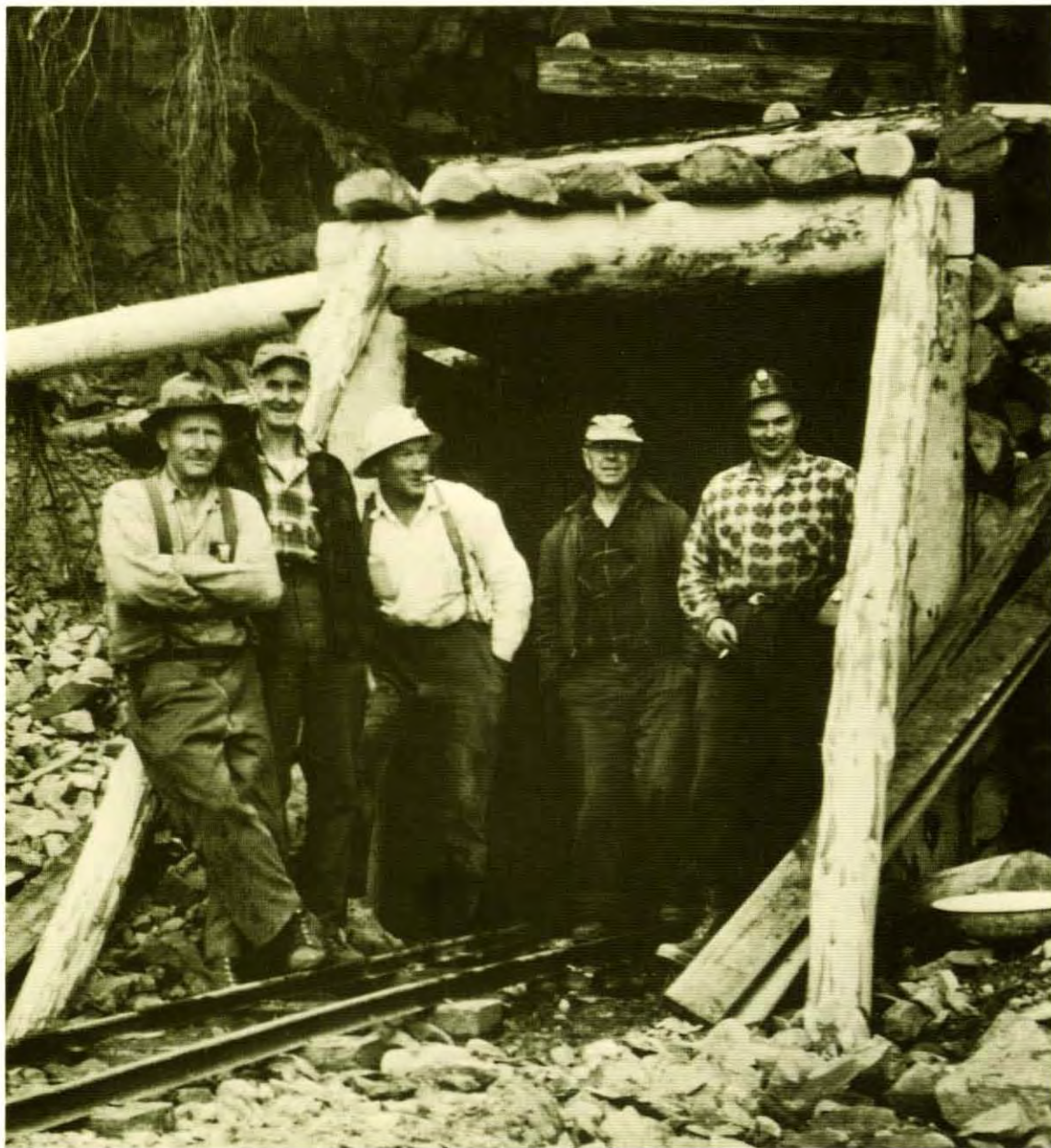
#16 portal retimbering and crew at the 5500 foot elevation.
