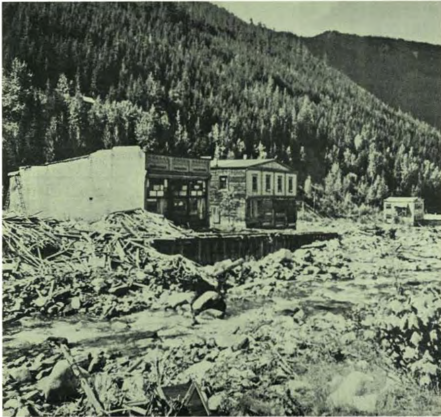
A plugged flume carrying the waters of Carpenter Creek through the centre of Sandon was responsible for the flood that carried away and destroyed many of the buildings.
