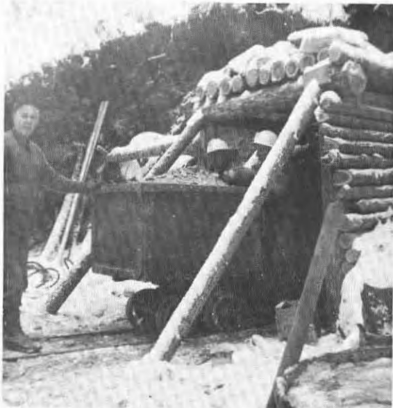
Ore car at Portal Annis Mines Ltd.
