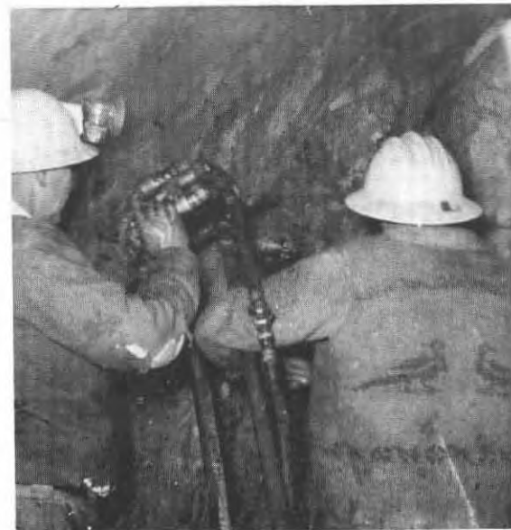
Drilling at the face in the tunnel.
