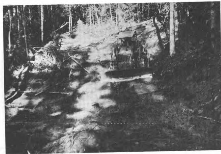
Bulldozing a trench at Annis Mines Ltd.
