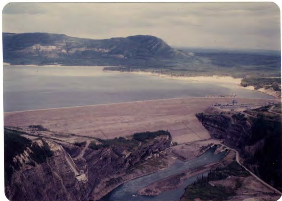
W A C Bennett Dam
