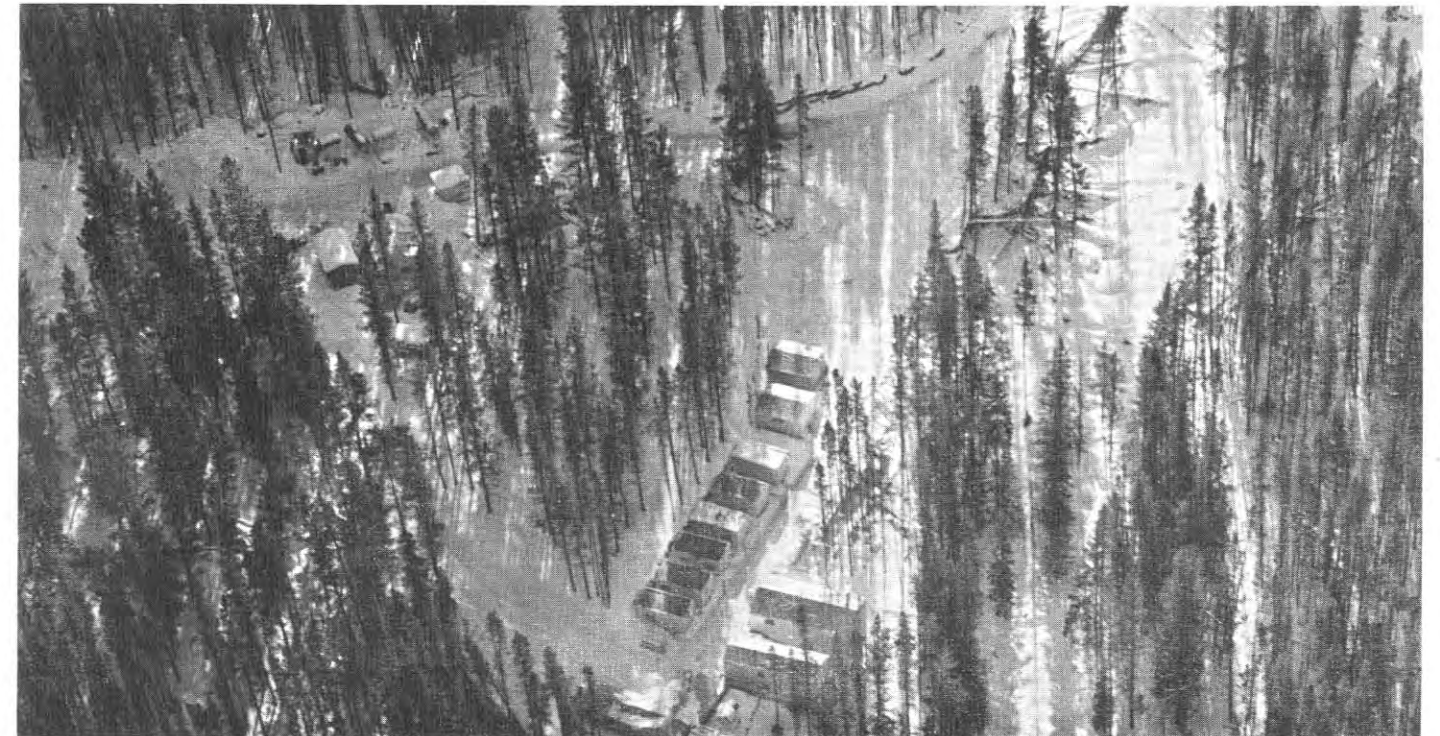
Highmont Campsite in Highland Valley with accommodation for 40 men.
