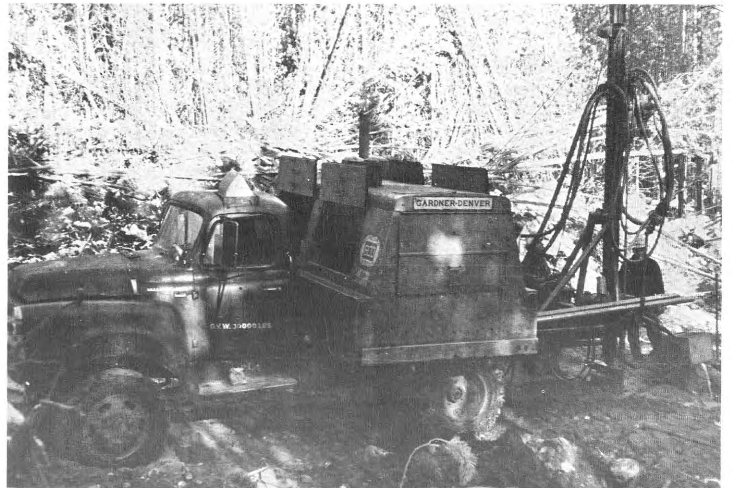
Truck mounted percussion drill rig (specially designed by COPCO) for the Highmont property.
