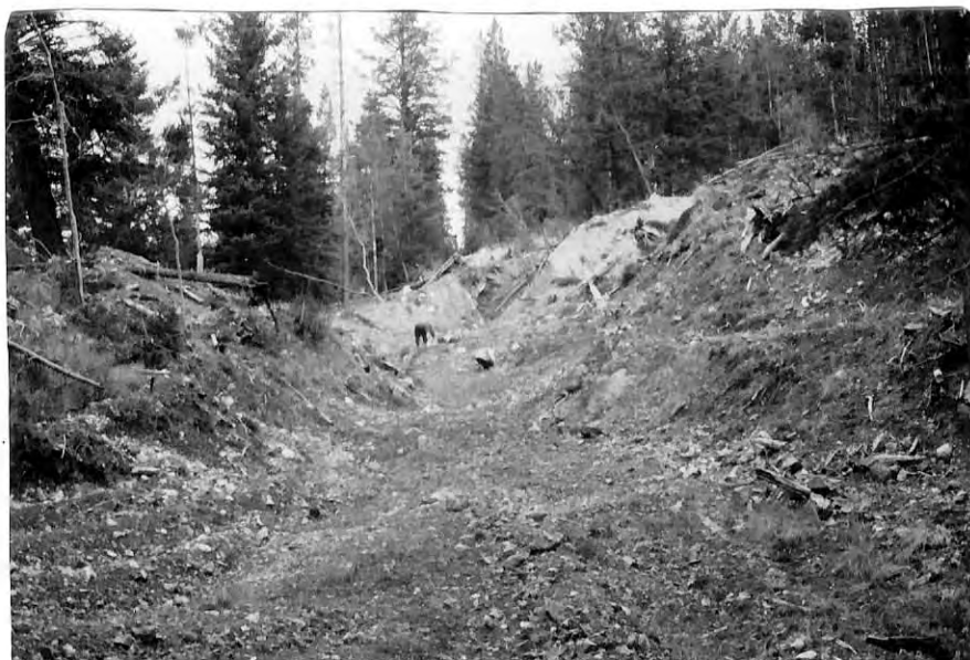
North-South trend in southern part of mineralized area exposes altered bedrock over 300 feet.
