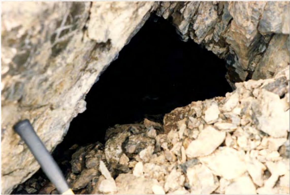
- partially caved adit below sample site C8R67R.
