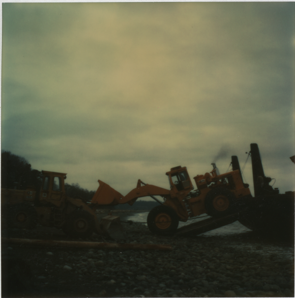
UNLOADING No. 1 AT PRODUCERS
